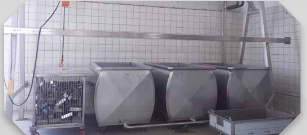
► Kaşar Kalıp Yıkama / Kashar Mould Washing
